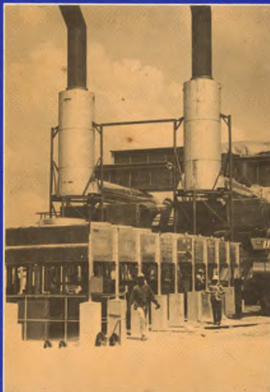
New Power Generating Plant - Garden of Eden
